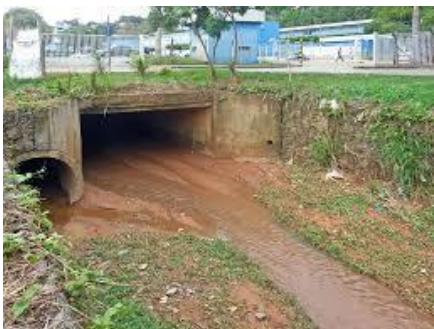
Canalization of Ribeirão Caladinho in Unileste, Coronel Fabriciano MG.
