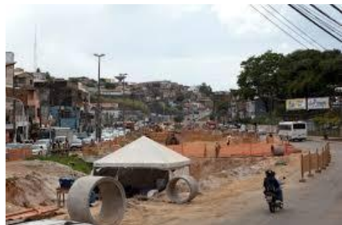
Drainage works on Avenida Vasco da Gama, Salvador.
